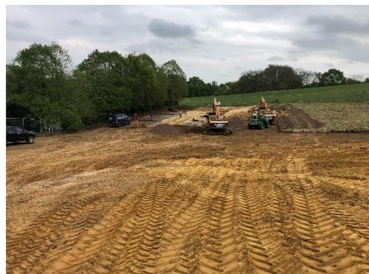
To enable the land to be transformed into their requirements, I was determined that the entire field would need remodelling which involved the movement of over 5000m<sup>3</sup> of soils some of which was used to fill some of the site, whilst the remainder had to be disposed of off site, fortunately the tests carried out on the soils before work commenced confirmed that the soil was mostly sand based and
